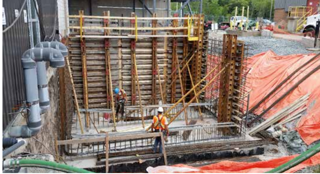
New Aerotech WWTF treatment process tankage under construction
